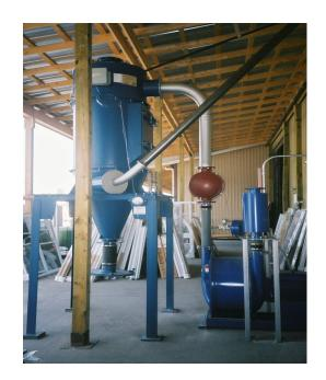
The installed system is presently collecting over 7.5 cubic feet of drywall dust from power wand sanders, sawdust from routers and circular saws every 12 hours of production time. Systech Design, Inc. was awarded the "sole source" contract for both systems because of our ability to provide a single point responsibility, including not only a complete engineering design package with all equipment and installation, but a 24/7 maintenance and service package.
