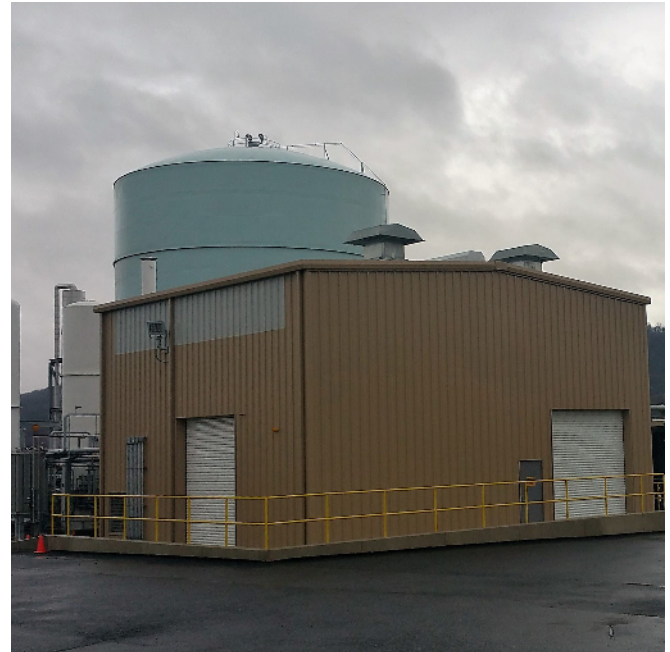
The two hoods located on the roof constitute the exhaust fans of the Rapid Purge System.
