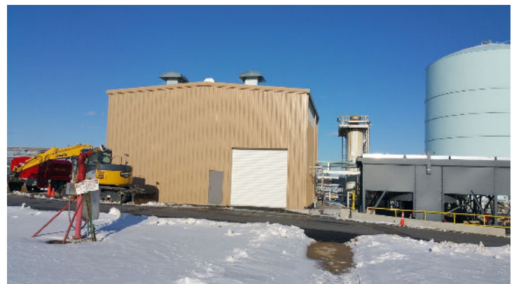
The tan steel building shown, houses both compressors with compressor coolers located outside.
