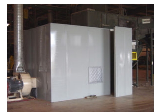
Rigid metal noise enclosure surrounding the hammermill that resulted in a 19 dBA reduction of noise levels within the facility.
