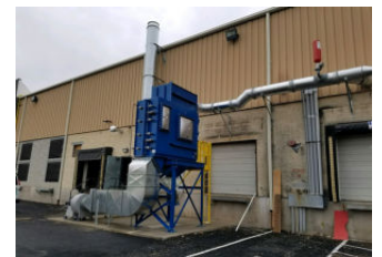
Donaldson Torit Model DFE 4-16 dust collector handling a hybrid mixture pictured with explosion venting and isolation suppression system installed.
