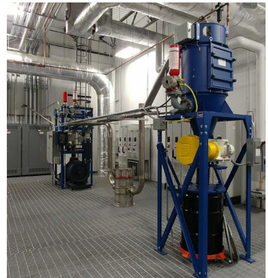
Donaldson Torit TD-182, airlock, HEPA filter housing and control panel
