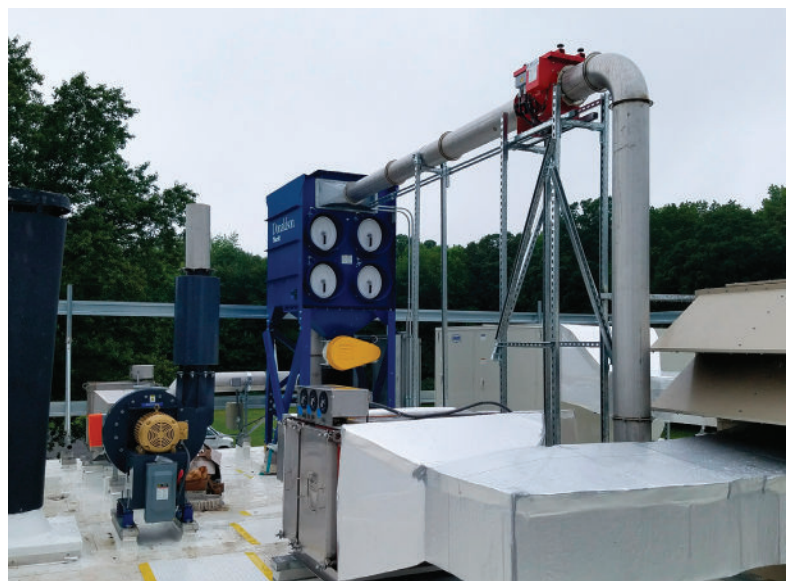
Spice blending application using a Donaldson Model DFO 2-8 dust collector, fan, silencer, rotary airlock and chemical explosion protection system.
