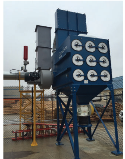
Donaldson Torit Model DFE 3-18 Dust collector with explosion isolation on spice grinding mill.
