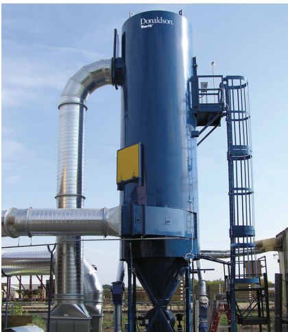
RF DUST COLLECTOR
