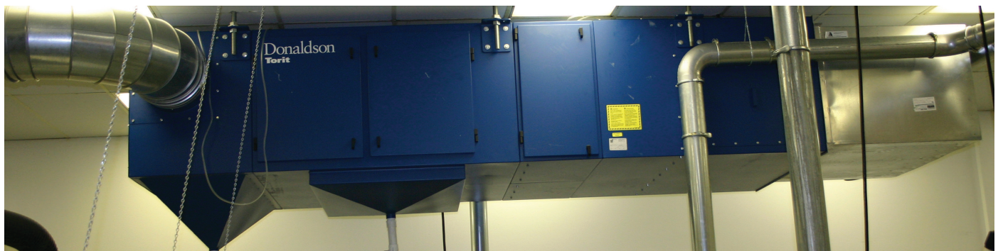
MODULAR MEDIAFILTER™ on Grinding 2,000 cfm ( 3,397 m 3 /h)
